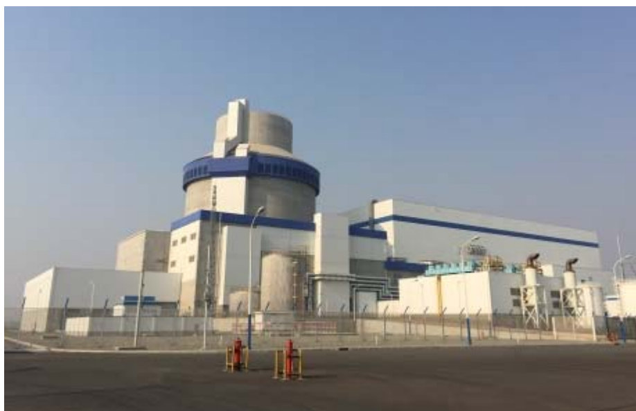
Haiyang unit 1 (Image: Westinghouse)
