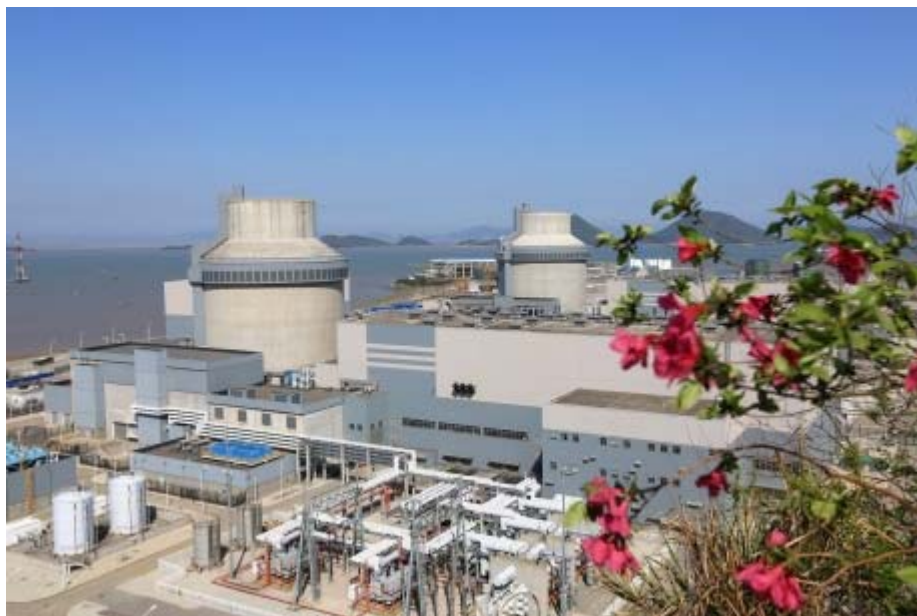
Sanmen units 1 and 2 (Image: Westinghouse)
