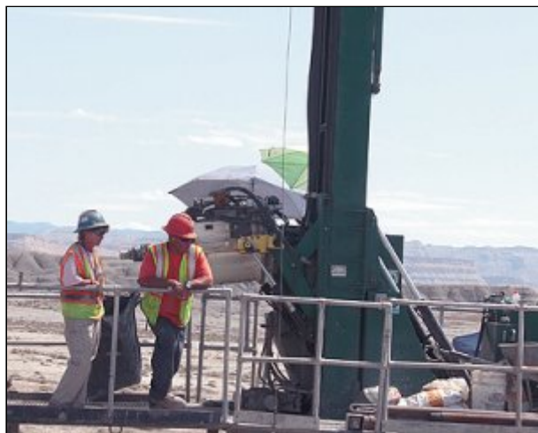
Drill rig operators collect soil samples.
