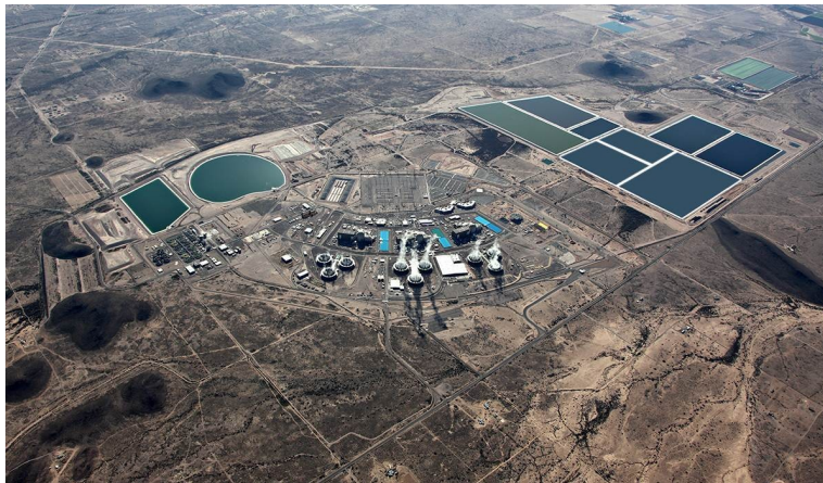
The Palo Verde Nuclear Power Plant in Arizona is the largest power plant in the U.S. by net generation. Source: AMWUA
