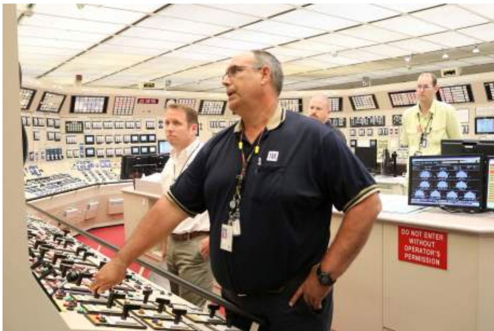
Reactor operator Bill Hahn synchronizes Watts Bar 2 to the TVA power grid (Image: TVA)
